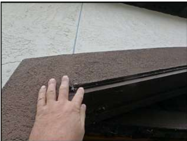
Head flashing installed at garage door per industry standards; typical
