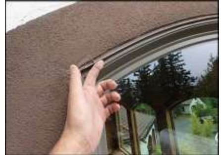
Head flashing installed at window; typical
