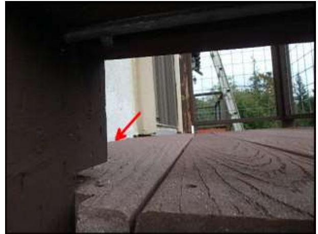
Flashing installed at deck ledger per industry standards (E4-F4)
