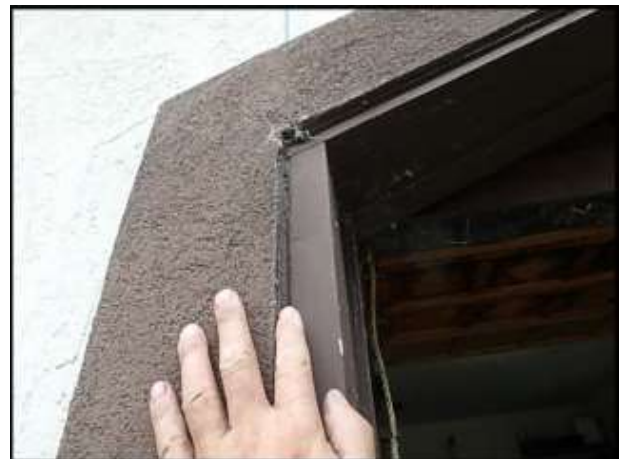
Sealant joint performing at garage door jambs; typical
